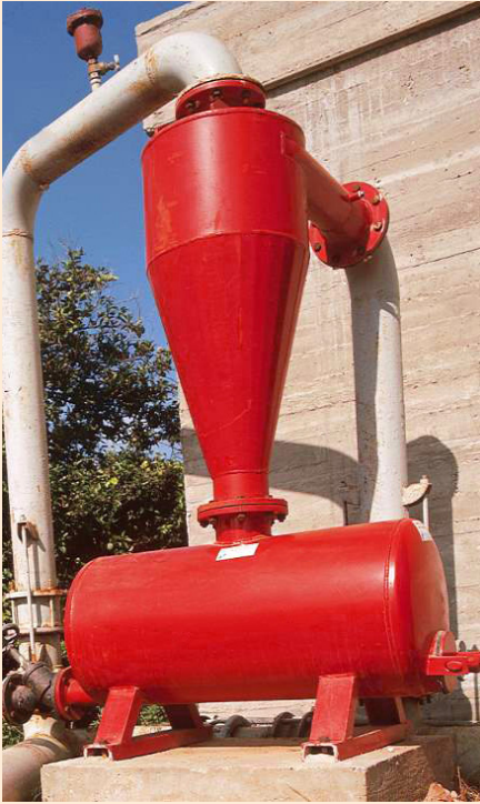
FIGURE 22. Separator/cyclone filter. (Courtesy of Netafim USA.)
